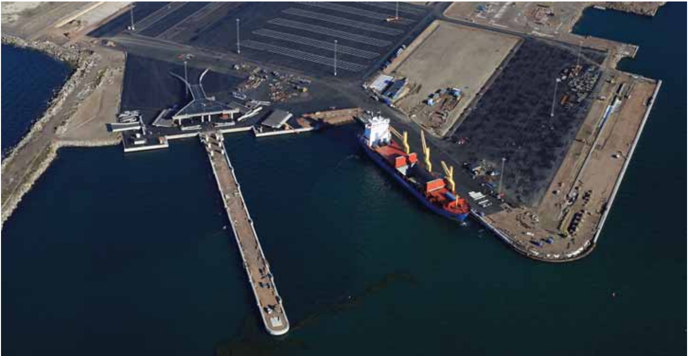
Part of Norra Hamnen where the RoRo ramp is under construction
