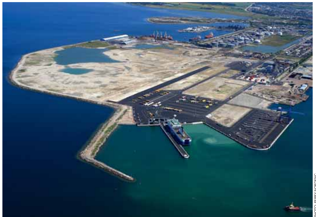
The Northern Harbour with the RoRo terminal in the foreground and the container terminal to the right.
