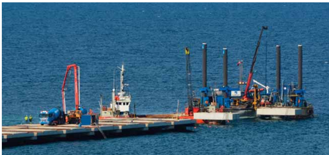
The quay deck, a concrete structure in 19 parts, was hoisted into place in April 2017.
